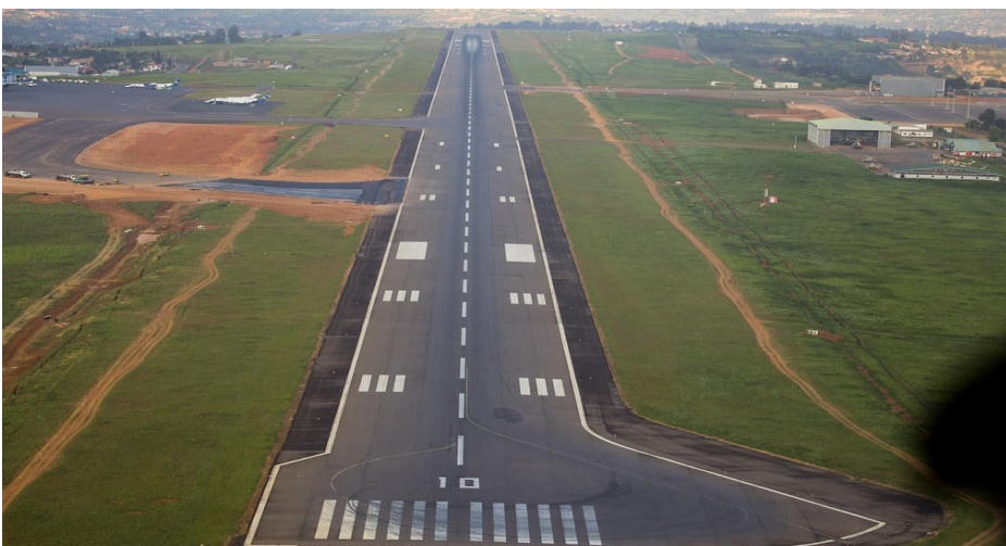
Runway, Kigali International Airport
